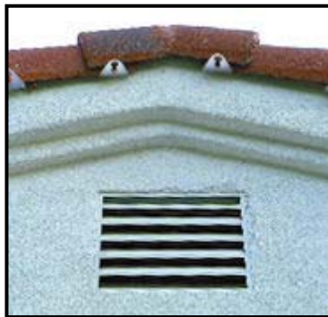
Figure 24. Double Fascia Covered by Stucco
